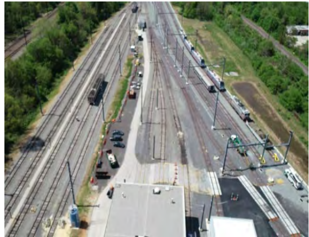
West end of Frazer Yard new storage tracks
